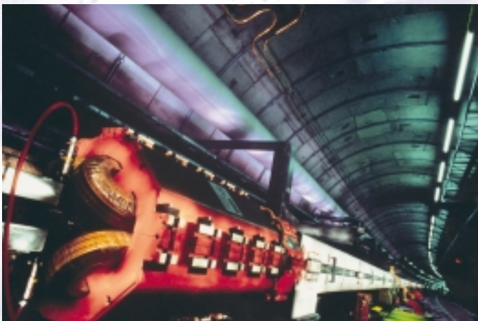
Blick in den HERA-Tunnel am DESY in Hamburg.
