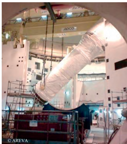
Fig. 5: Introduction of the second Steam Generator into the Reactor Building at Flamanville 3 EPR reactor, France.
