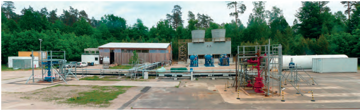
Fig. 5: Surface installations at the geothermal research platform Groß Schönebeck with production well (red), injection well (blue), function hall (rear left) and ORC-plant with cooling towers (rear right).
