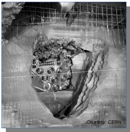
LEP Tunnel break through, 1986
