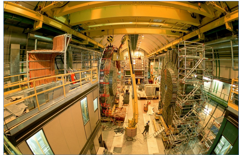
Dismantling of the DELPHI detector at LEP (source: CERN/CDS)
